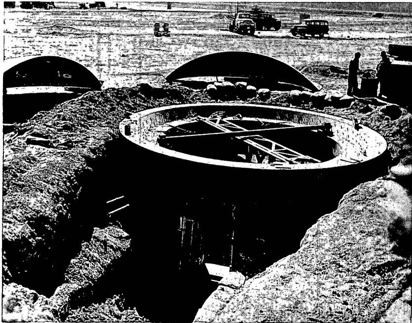
Fig. 9—Foundation for aluminum dome. Two halves of shell are in background.
